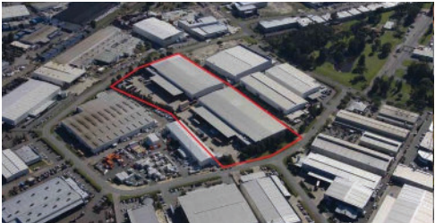
7-11 & 25-27 Gauge Circuit, Canning Vale
