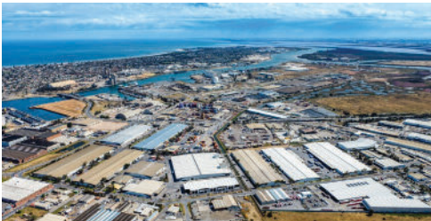
Port Adelaide Distribution Centre, Gillman
